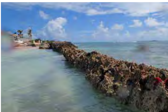
PHOTO 7: ROCK FORMATION ACTING AS TERMINAL GROIN
